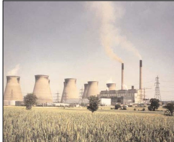
Ferrybridge Power Station, UK
